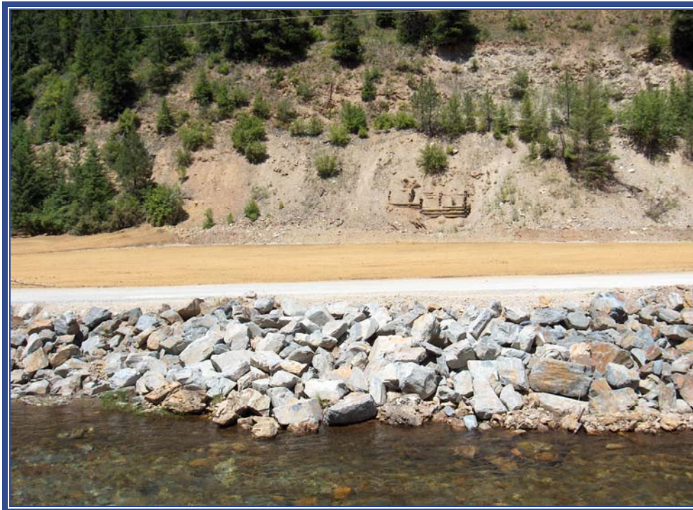
Golconda - Post Remediation
